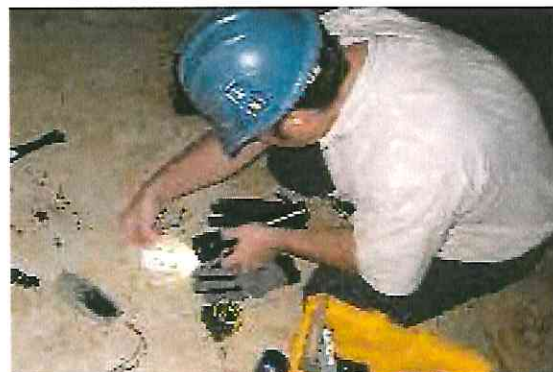
CSI determines the reason for your coating failure by conducting a detailed and thorough on-site investigation and methodical assessment.
