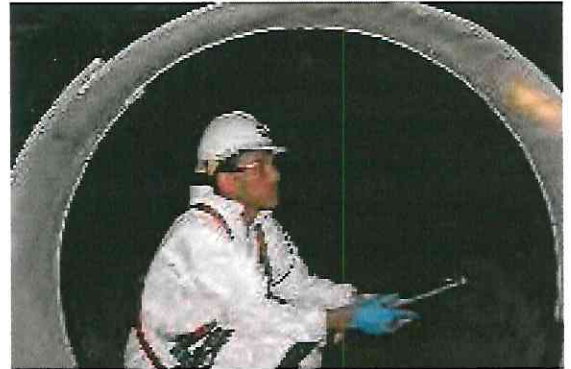
Skilled inspectors scrutinize PVC liner welds and seams to determine proper installation.
