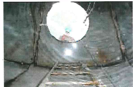
CSI's team of divers and engineers use advanced technology to inspect your reservoir and make repairs without having it drained.
