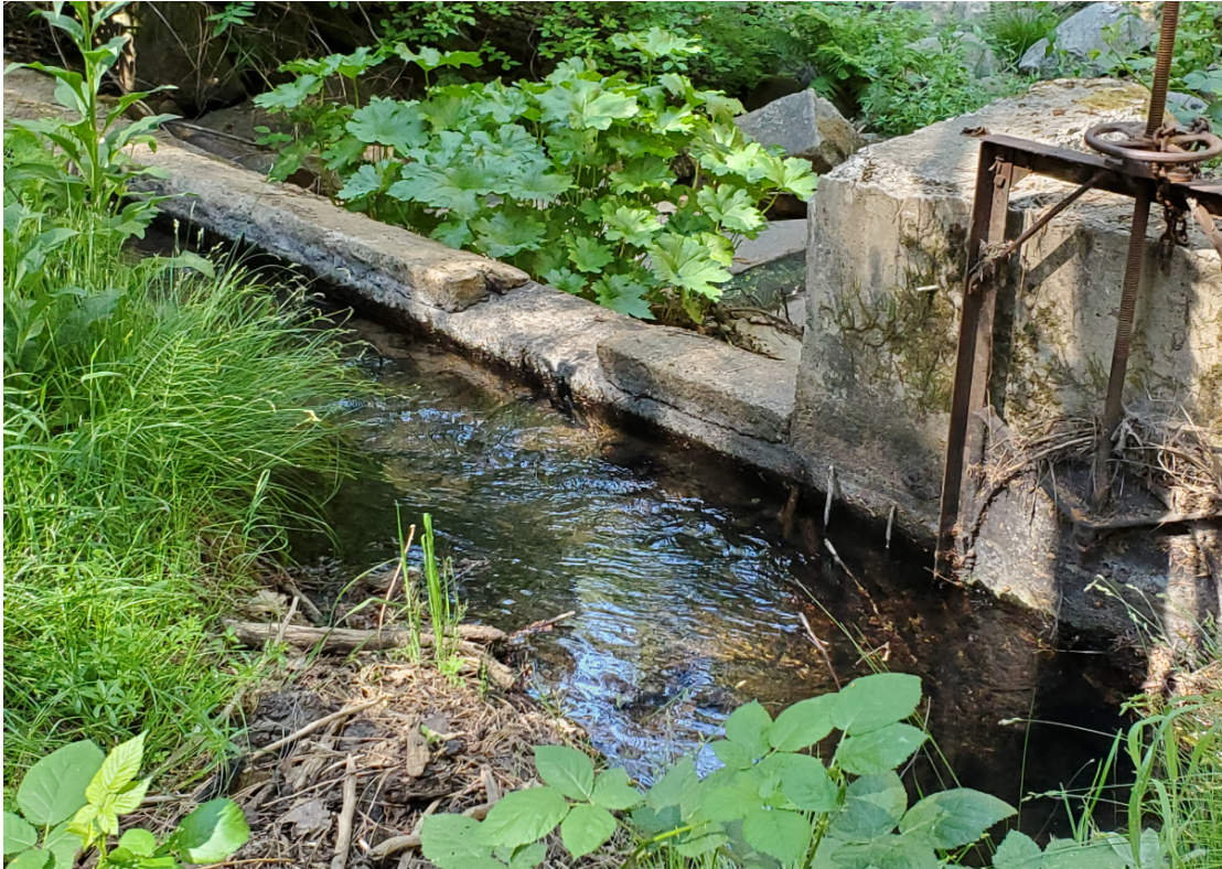
Figure 5. Bear Creek Diversion
