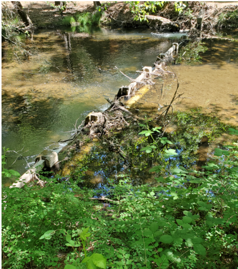
Figure 7. CCWD Middle Fork Pumping Plant
